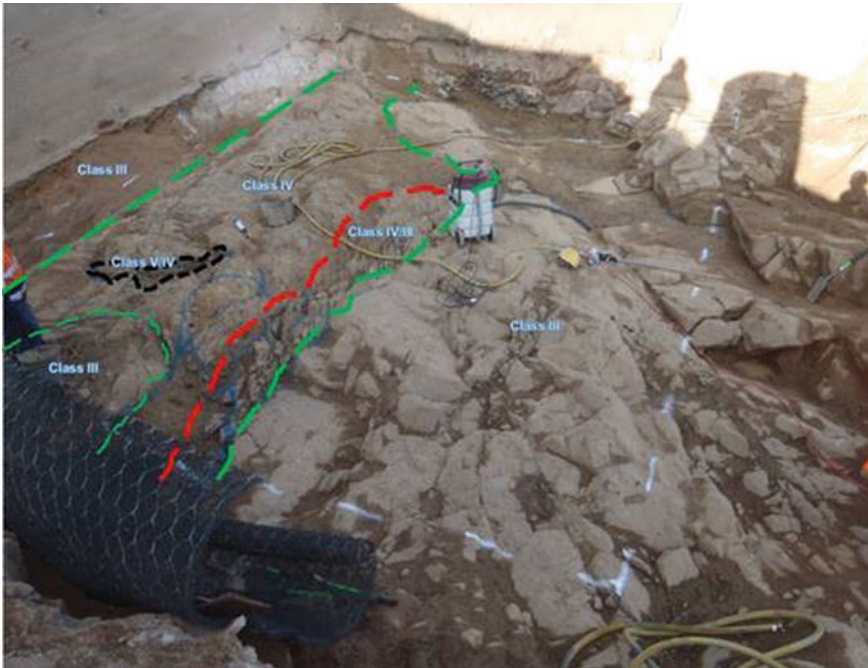
Fig. 16 Exposed rock at elevation of RL 849 m at Pier 2
