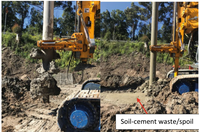
Fig. 17 WSM construction rig and produced recycled soil–cement waste
