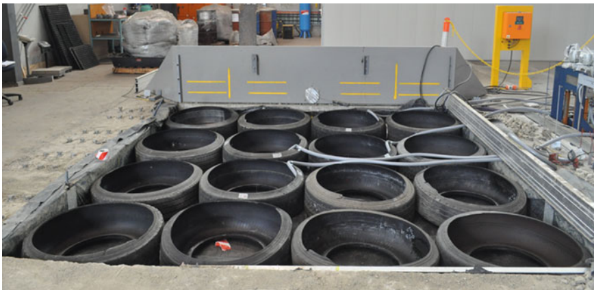
Fig. 23 Tyre cell assembly placed for the preparation of capping layer
