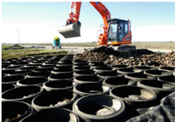
Fig. 13 Placement of tyre cells in the field application
