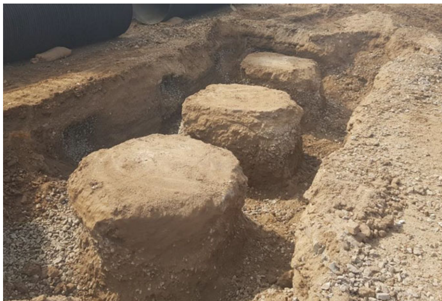
Fig. 16 Exposed column head of WSM columns at 1.1 m depth
