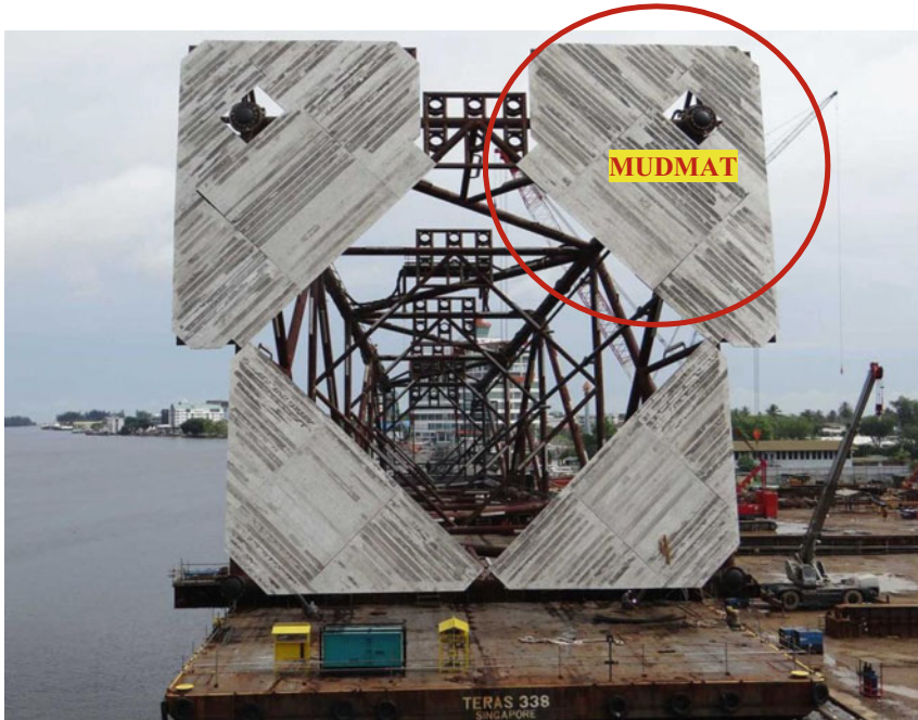
Fig. 3 Mudmat for jacket structure
