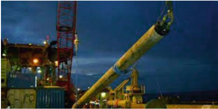
Fig. 5 Pile lifting & handling [10]
