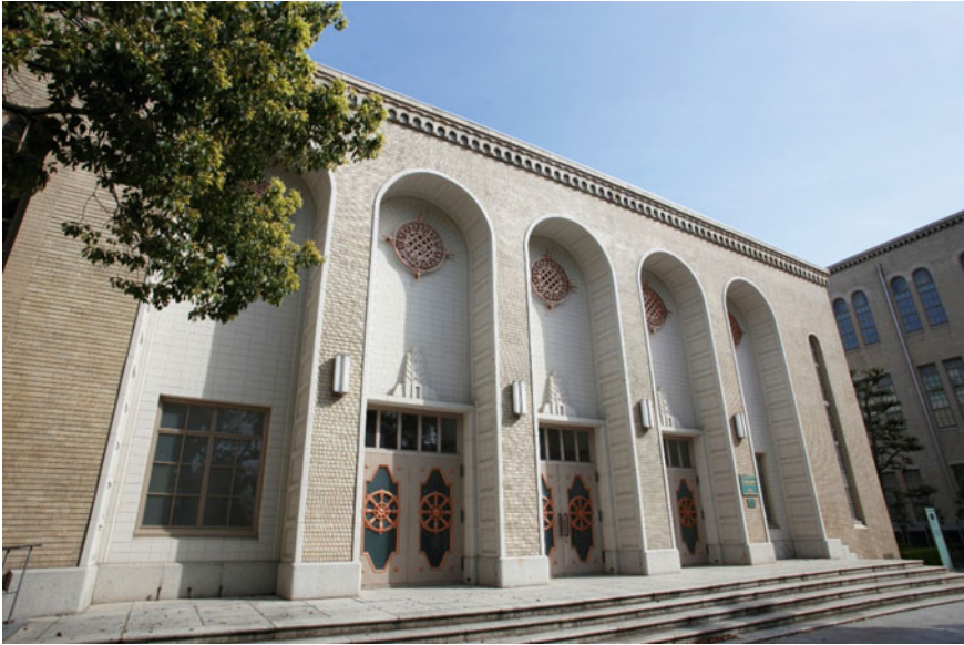
Photo 9.3 Rokkodai Auditorium (Idemitsu Sazo Memorial Rokkodai Auditorium), standing on the Rokkodai Campus, a National Registered Cultural Property (built in 1935).
