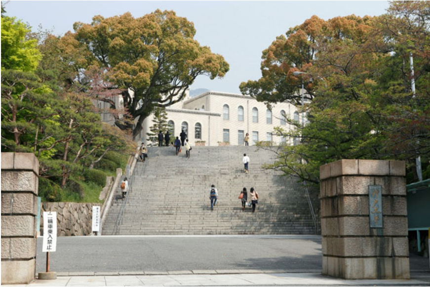
Photo 12.1 Looking toward the Rokkodai Main Building from the main gate of Kobe University
