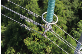
(a) Nuts are not properly installed
