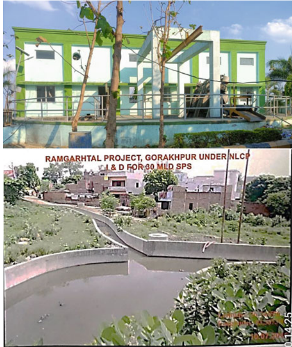
Fig. 17.8 STP in Ramgarh Tal lake, Gorakhpur, UP
