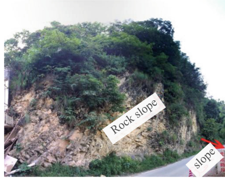
Fig. 3. Inner rock slope of highway
