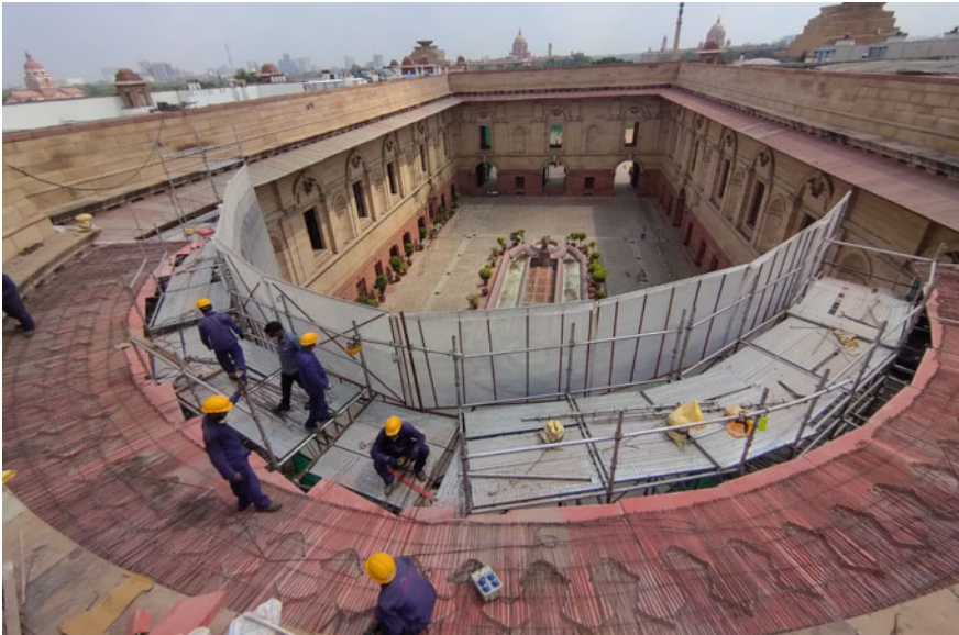
Fig. 31 FRP formwork installed and additional reinforcements anchored
