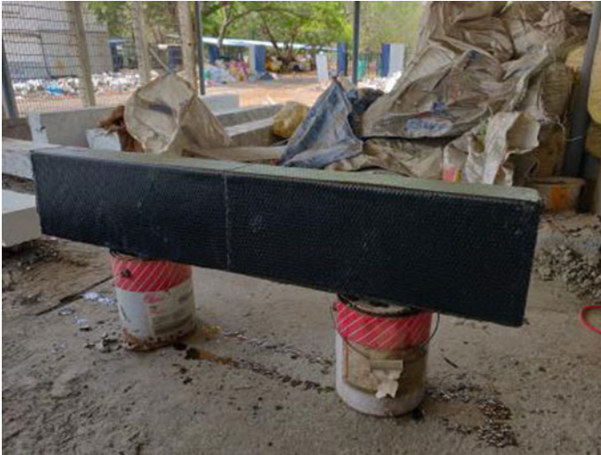
Fig. 7 CFRP laminate installed to the beam using the EBU Method
