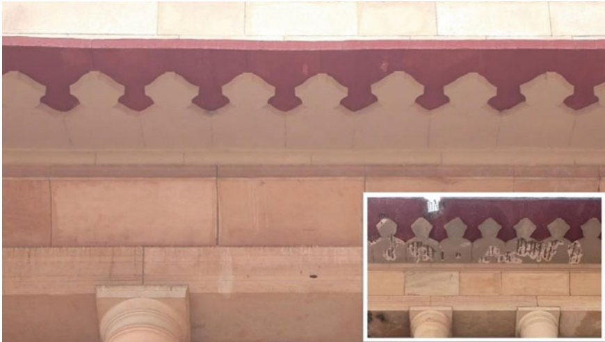
Fig. 32 Photos taken before (inset) and after retrofitting the chajjas of Rashtrapati bhavan
