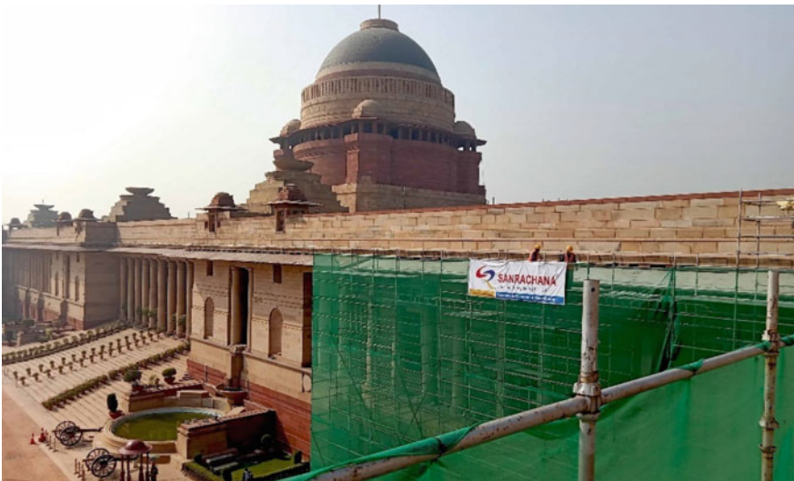
Fig. 26 The front portion of Rashtrapati bhavan photographed while retrofitting was underway
