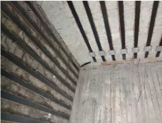
Fig. 22 Prestressed (top) and non-prestressed (side) carbon laminates, inside hammerhead
