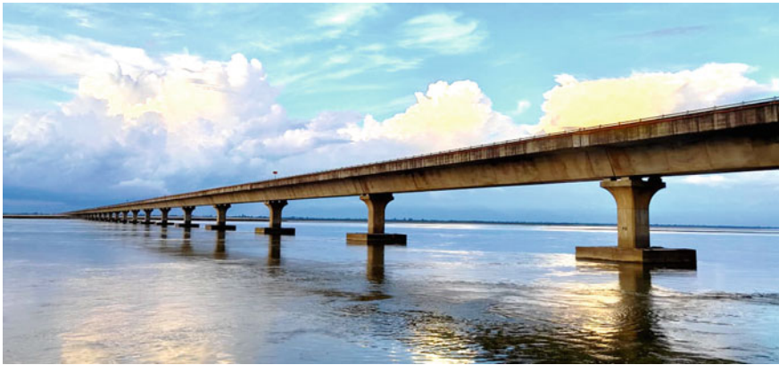
Fig. 13 Photograph of the Assam bridge taken before retrofitting
