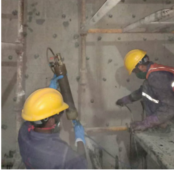
Fig. 21 Pressure grouting on vertical walls from inside the hammerhead
