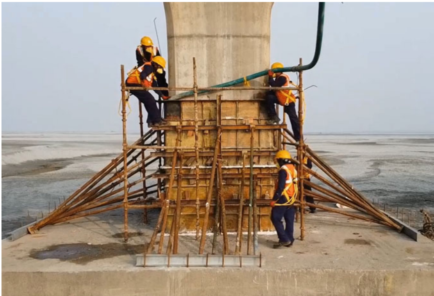
Fig. 16 Protection of the FRP wraps on the pier using micro-concrete jacketing
