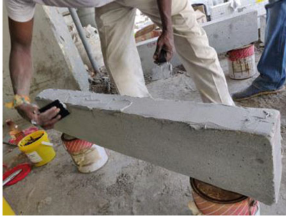
Fig. 5 Applying Epoxy adhesive for installation of CFRP
