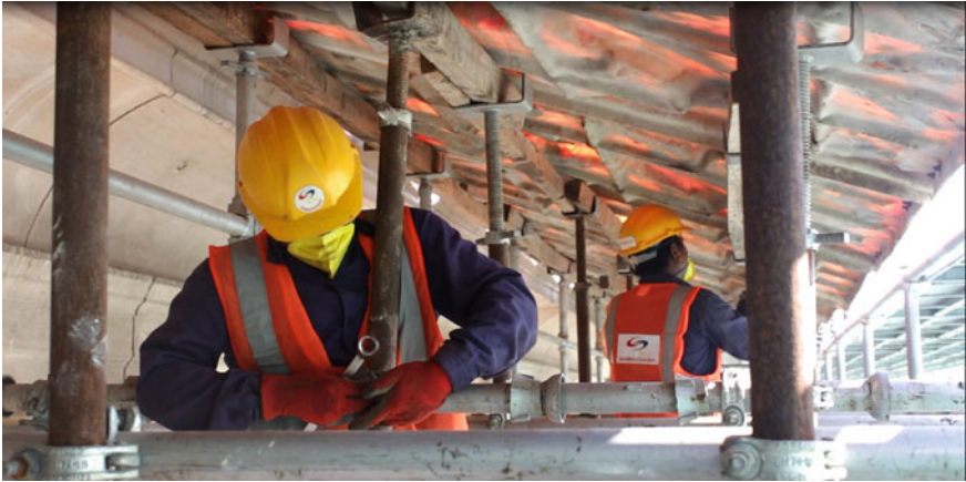
Fig. 30 FRP formwork installed for light-weight concreting, after demolition of existing chajja
