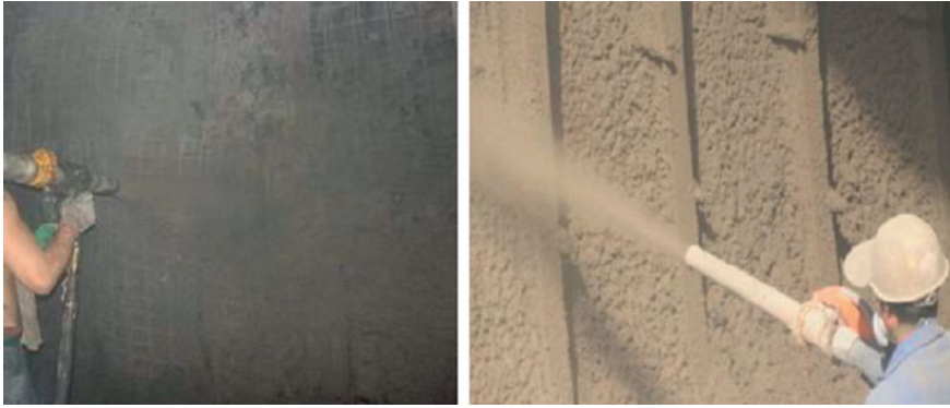
Fig. 18 Shotcrete in RC walls and tunnels [106]
