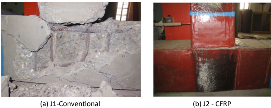
Fig. 16 Failure pattern noticed in the joint specimens
