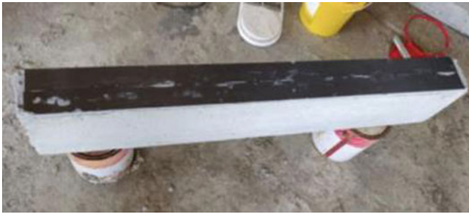
Fig. 6 CFRP laminate installed to the beam using EB Method
