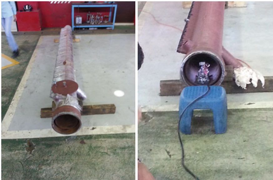
Fig. 59.4 Robot with the image acquisition system is tested on a real specimen of the boiler header in SJSI to verify the results tested previously in the lab
