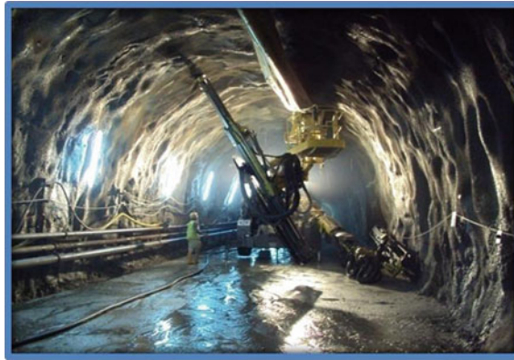
Fig. 1 Excavation of NATM I at Pahang-Selangor raw water tunnel
