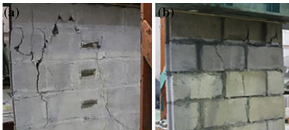
Fig. 9 Crack observed in the wallette test; (a) 15 mm mortar thickness and (b) 10 mm mortar thickness
