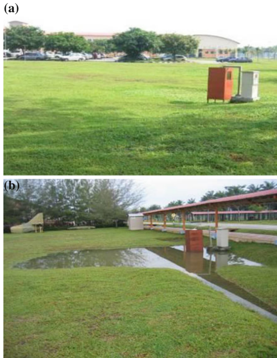
Fig. 4 Dry detention pond in the Engineering Campus of USM (Penang) [8]. a Before storm event—as football field. b After storm event—as temporary water pond
