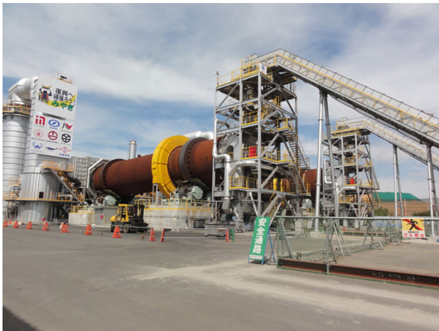
Photo1 Disposal facility for disaster waste (Ishinomaki-city, Miyagi prefecture)
