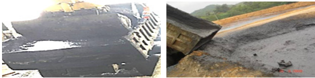
(a) Mixture of heavy metal materials and solidified products at tipper lorry. (b) Final disposal of cementation product at reserve area in secure landfill.
