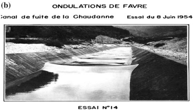
Fig. 5 a from [5]. b Tests of release in Chaudanne HP station (France), courtesy Electricité de France
