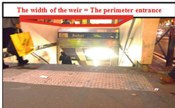
Fig. 1 Schematic representation of the configuration of the spillway formula for emergence of type outlet staircase by DHI office
