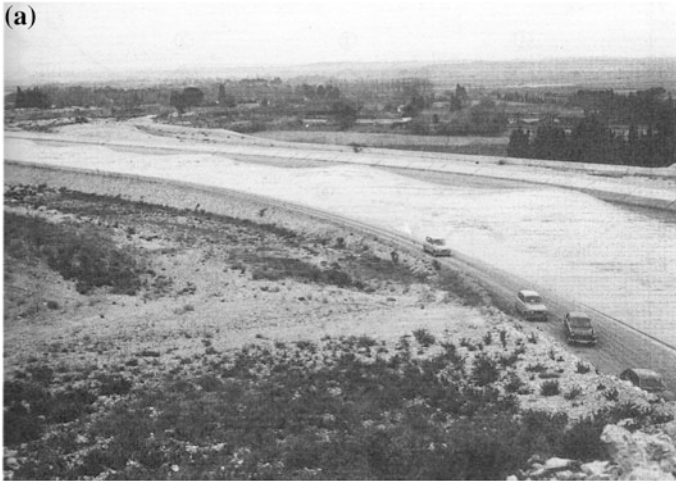
Fig. 6.10. Advancing undular surge in a Durance River (France) power canal (courtesy Electricité de France)
