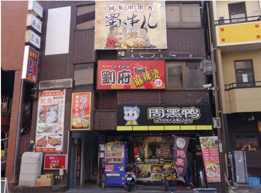
Fig. 3.10 Multi-tenant building with three Chinese restaurants near Nishi-Kawaguchi Station in Kawaguchi City. Source Taken by the author in 2018
