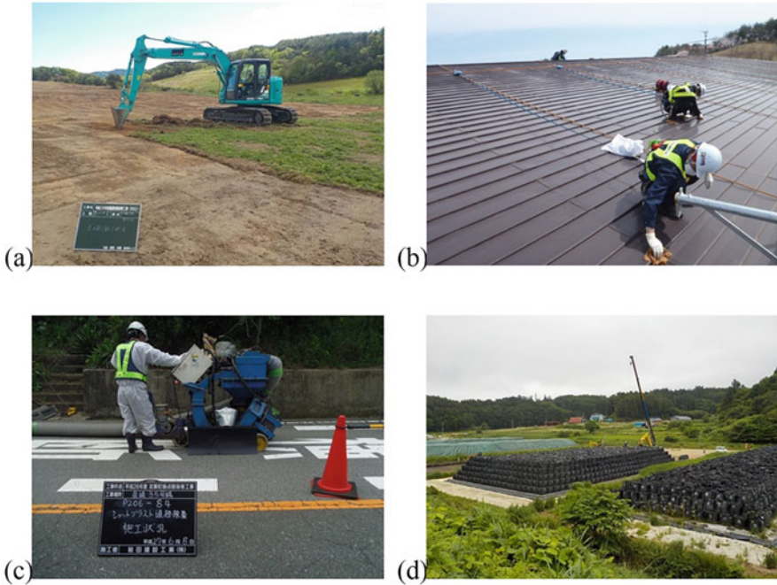
Fig. 3.10 Decontamination process in Fukushima: (a) grassland (IT-01-P0041), (b) roof and buildings (IT-01-P0034), (c) road (FB-01-P0012), (d) temporary storage site (IT-02-P0056). (Ministry of the Environment, Japan 2016)
