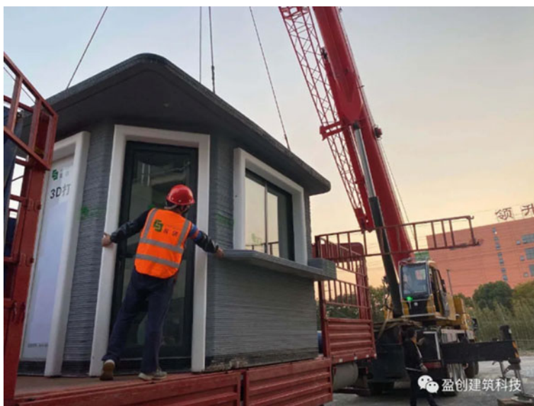
Fig. 5 3D printed quarantine booths (Guideline for Disinfection and Sterilization in Healthcare Facilities 2008)
