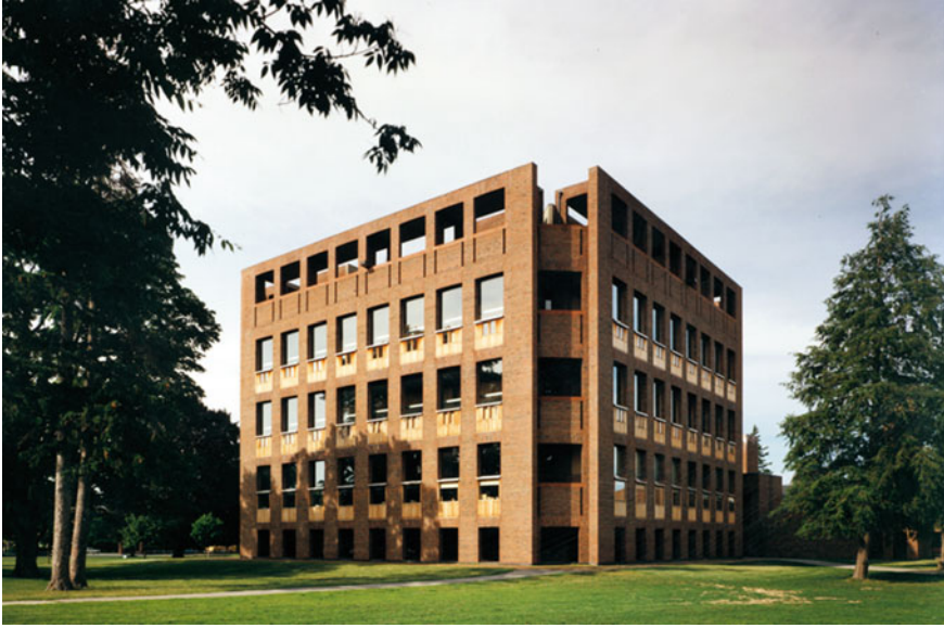
Fig. 4 Exterior view of the Philip Exeter Library, USA
