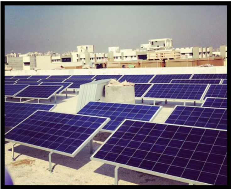
Fig. 22 Installation of solar panels on the terrace
