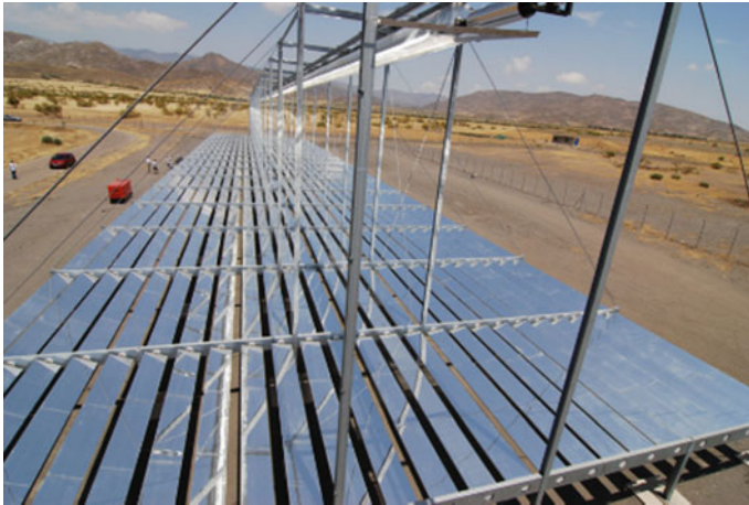
Fig. 2 Linear Fresnel reflector [25]
