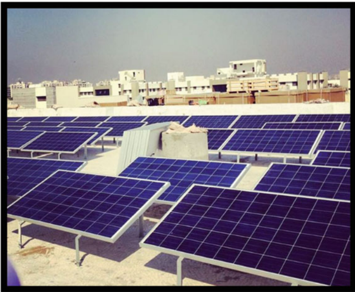
Fig. 22 Installation of solar panels on the terrace
