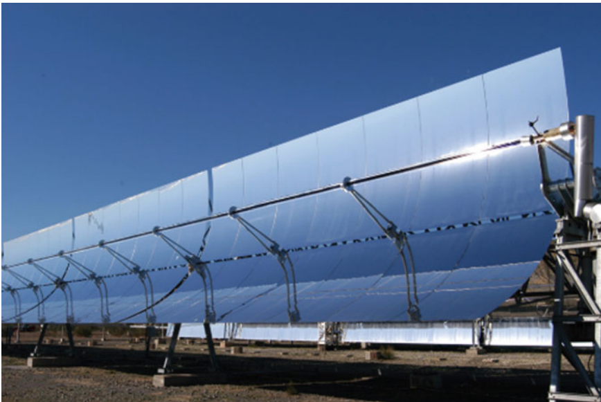
Fig. 1 Parabolic trough collectors [25]
