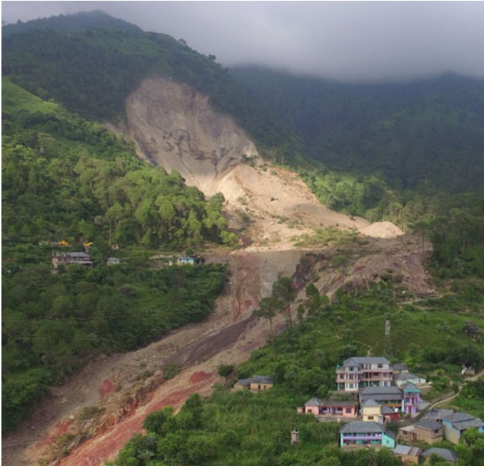
Fig. 1 (Left) Water-triggered Paddhar landslide in 2017 in Himachal Pradesh due to intense and persistent rainfall. The failed slope was approximately 250 m high and 150 m in width. Approximately 300 000 m 3 debris was displaced for approximately 950 metres resulting taking 46 lives (Courtesy Himachal Pradesh State Disaster Management Authority)
