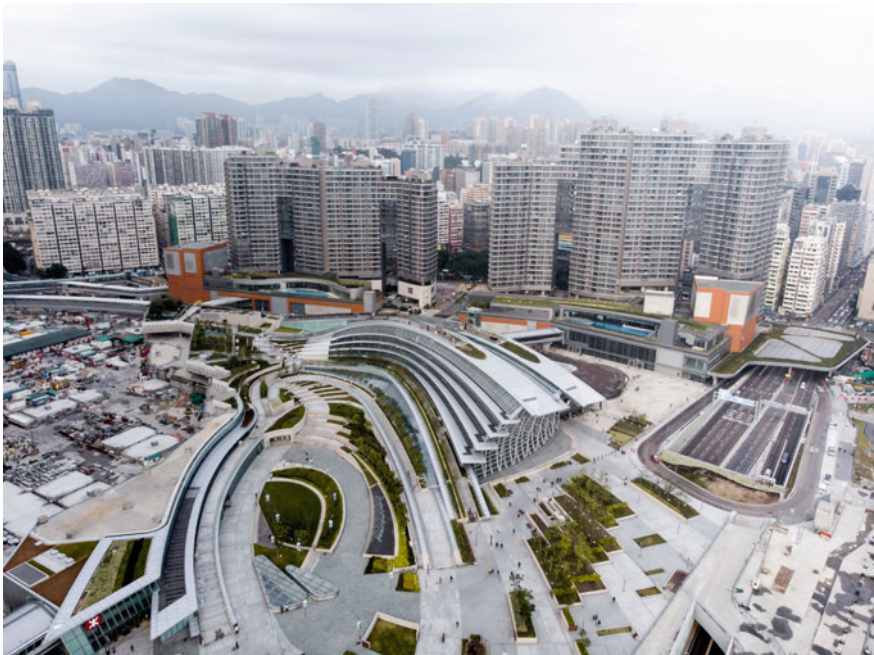
Fig. 6 Above: Aerial view of the West Kowloon Station (WKS), Station Entrance Building (SEB) and Civic Plaza. The WKS top-side Commercial Development provision is located on the northern-end of the Civic Plaza. Austin Station (Metro Station, standard box-type SEB) with top-side development (Residential usage) is sited in the background. Source Aedas (2020) [2]
