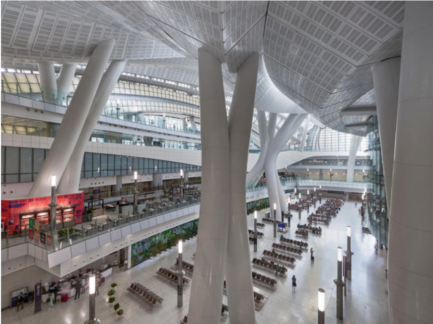
Fig. 7 Above: Interior of the West Kowloon Station (WKS), underside of Station Entrance Building (SEB), curved mega-columns supporting a free-form roof, allowing daylight to flood into the Departures Hall. Source Aedas (2020) [2]
