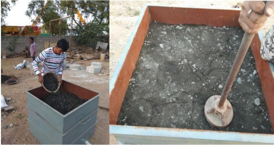
Fig. 5 Preparation of base course layer
