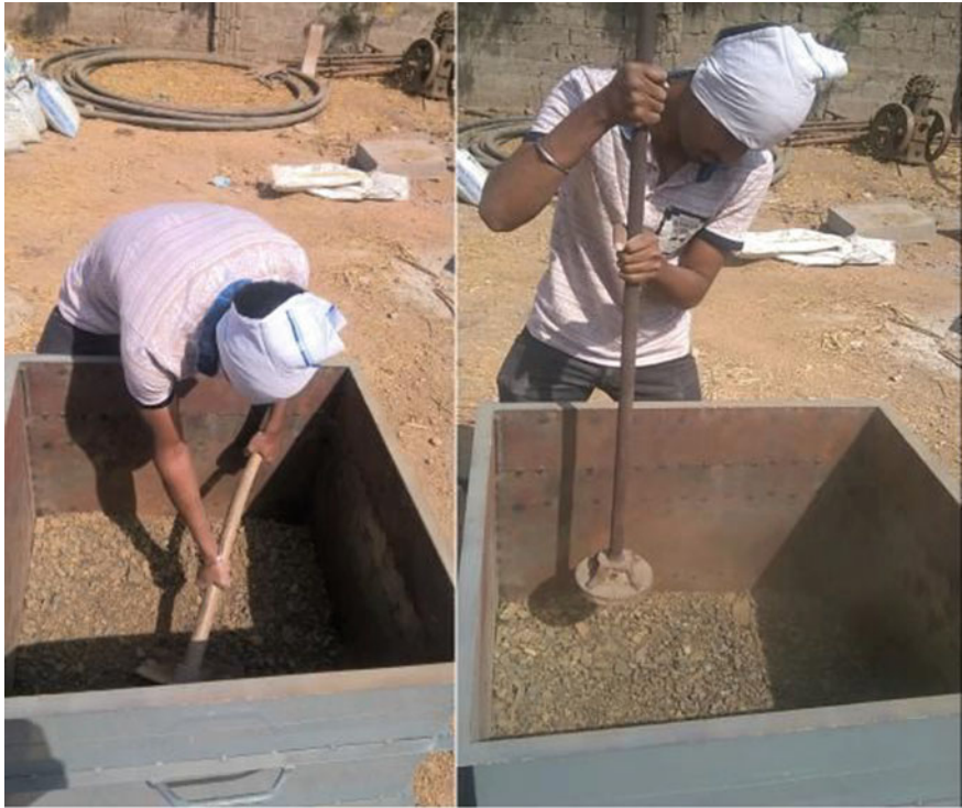
Fig. 4 Preparation of bottommost layer filling and compacting subgrade and granular subbase
