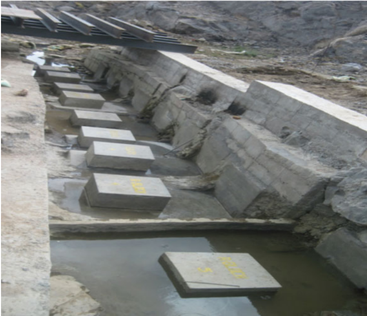
Fig. 3 Photograph of open trench excavation and shear test locations [10]
