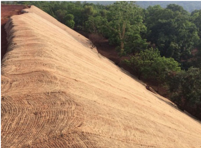
Fig. 2 Laying of JGT on slope surface
