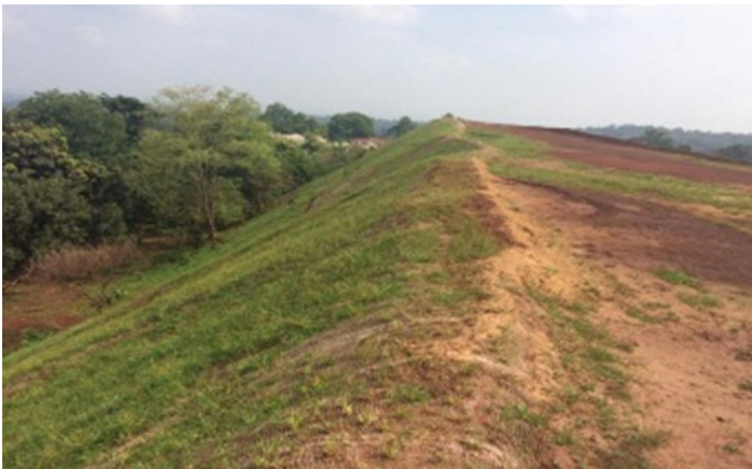
Fig. 3 Stabilized OB dump with growth of vegetation
