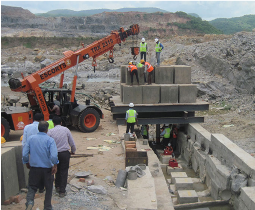
Fig. 4 Photograph of open trench showing Kent-ledge loading arrangement [10]
