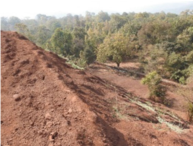
Fig. 1 Destabilized OB dump of slime
