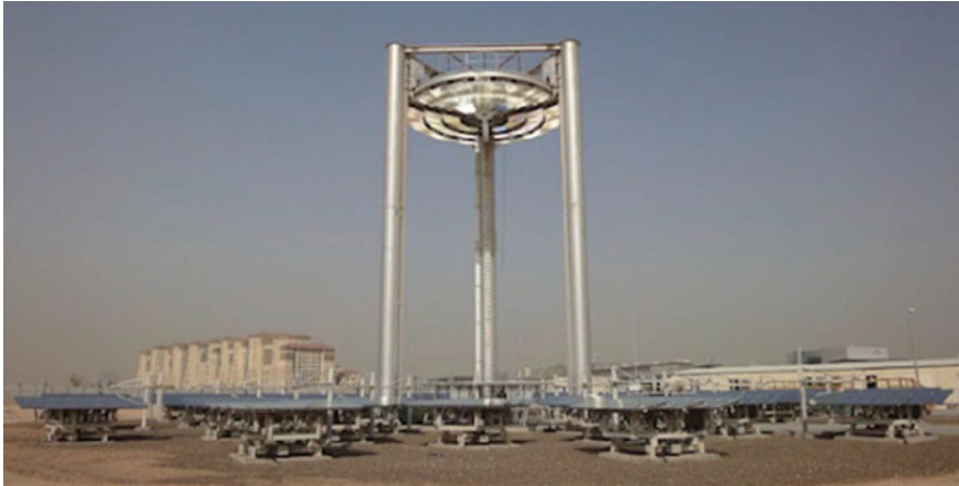
Fig. 3.35 Solar beam down concentrator facility at Masdar Institute Solar Platform (MISP) [53]
