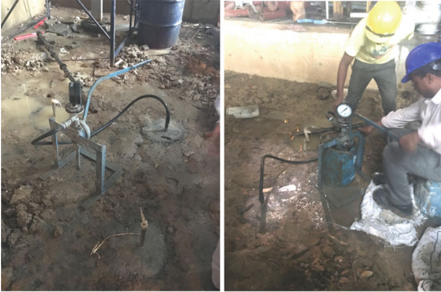
Fig. 5 Trial grouting in progress
