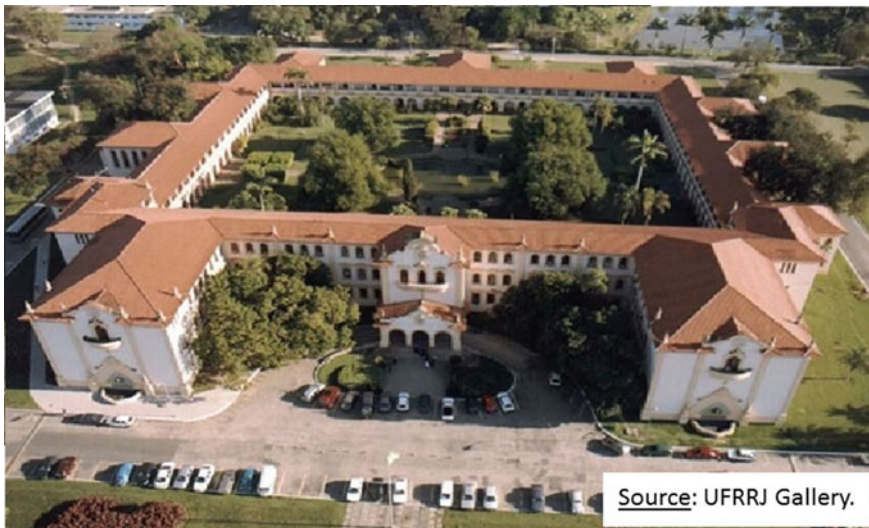
Fig. 3.14 Area View of Main Building—Federal Rural University of Rio de Janeiro/UFRRJ
