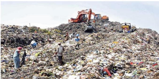
Fig. 1 Ghazipur landfill site
