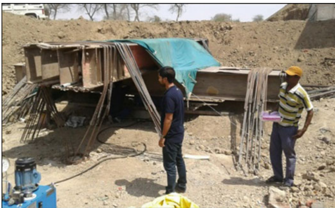
Photograph 2 Setup of vertical pile load test
