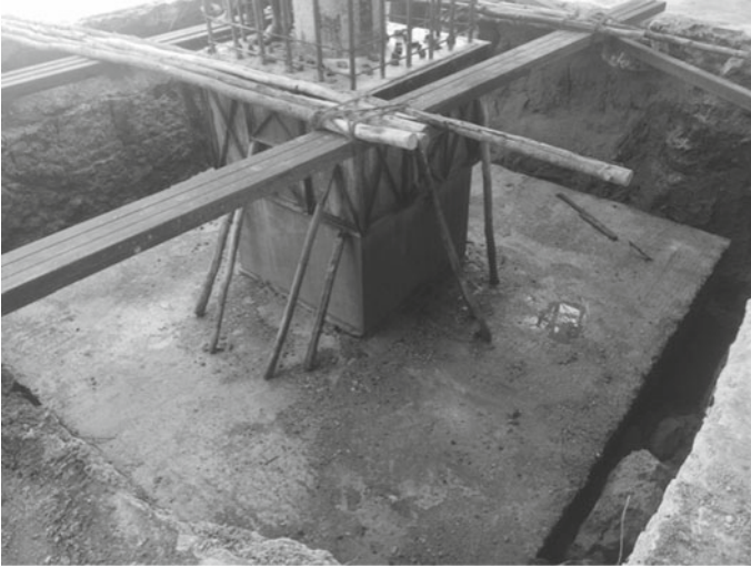
Fig. 6 Site photographs showing footing after concreting
