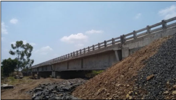
Photograph 4 Major river bridge
