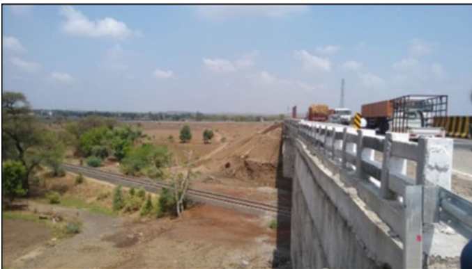
Photograph 5 Railway over bridge (ROB)
