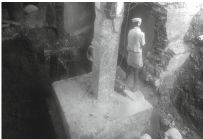
Fig. 4 Site photographs showing existing footing and underpinning before concreting
