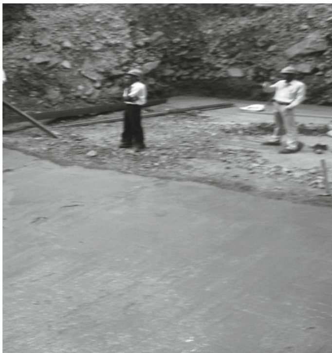
Fig. 6 Plum concrete laid in part area
