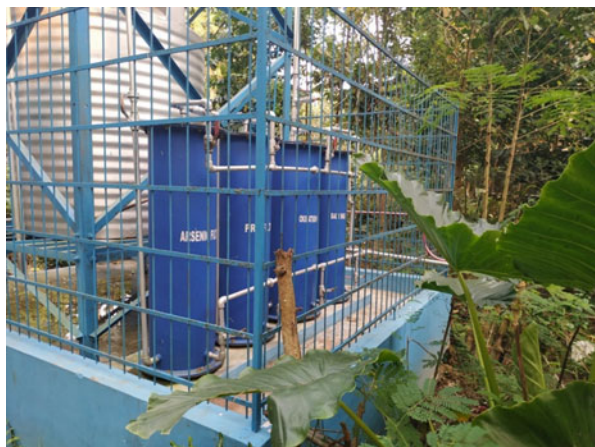
Fig. 8.6 Showing community level Arsenic removal unit by adsorption techniques in Deganga, block, North 24 Pargana, West Bengal
