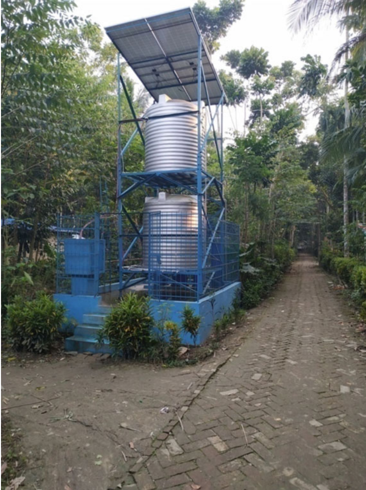
Fig. 8.5 Showing community level water filtration unit in Deganga, block, North 24 Pargana, West Bengal
