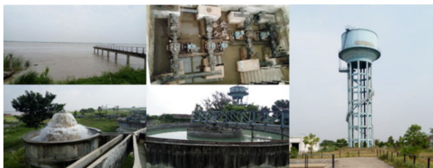
Fig. 7.19 Moujampur plant in Bhojpur District utilizing Ganges water for arsenic exposed population
