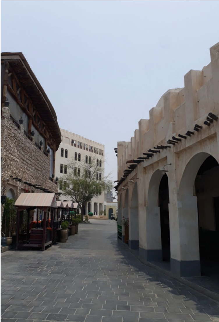
Fig. 5.7 Souq Waqif in Doha, after the restoration works (Credits: author)
