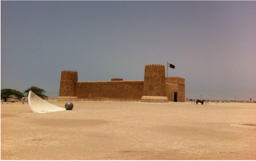
Fig. 5.1 Al Zubarah fort reused as a museum of the fort, after the completion of the restoration works (Credits: author)
