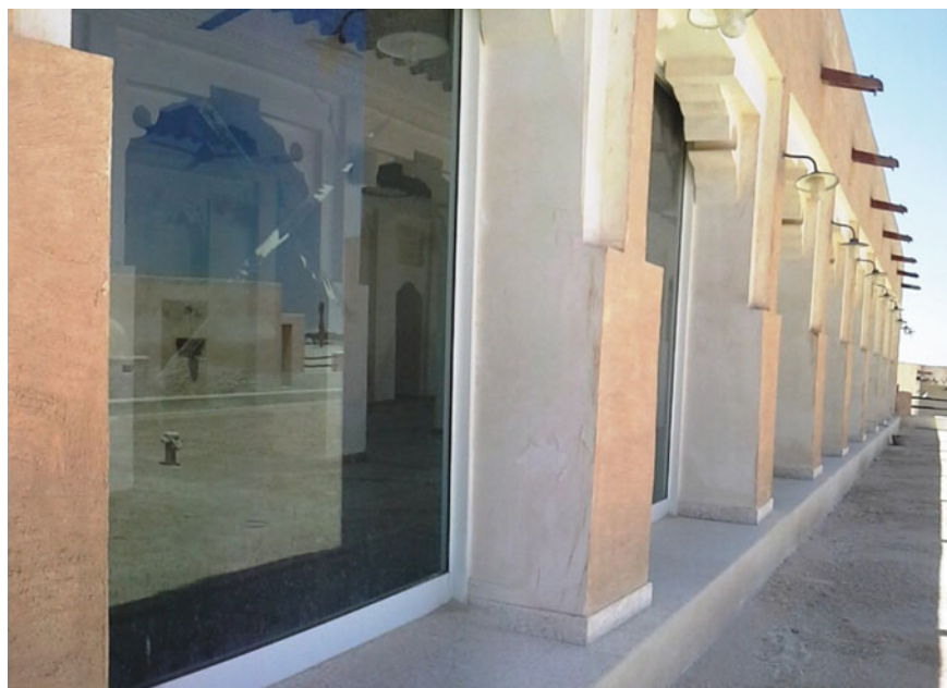
Fig. 5.4 Al Ruwais Mosque during the restoration works (Credits: author)
