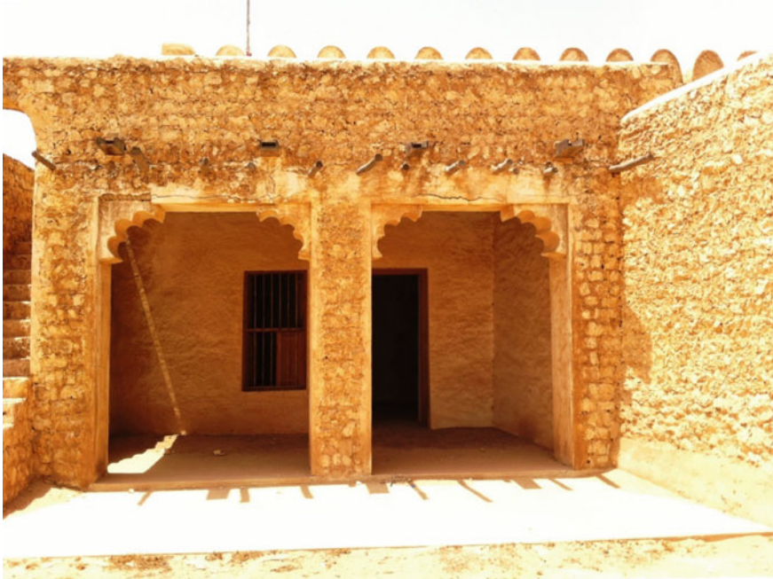
Fig. 5.2 Al Taghab fort in Qatar. Completed restoration works (Credits: author)
