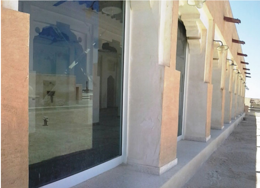
Fig. 5.4 Al Ruwais Mosque during the restoration works (Credits: author)
