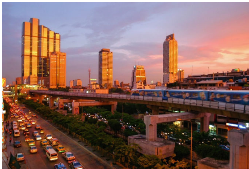
Fig. 4.2 Sky Train above the road system in Bangkok (Commons 2004)
