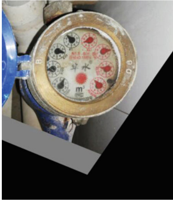
Fig. 2 Large dial after perspective transformation
