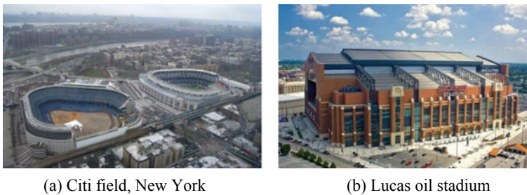
Fig. 2 Precast reinforced concrete structures of large-scale stadium
