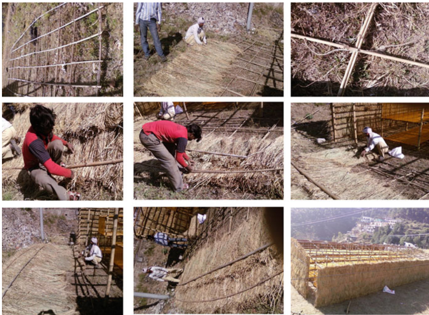
Fig. 12.6 Steps in preparation of mushroom growing shed in North India
