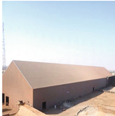
(b) Corrective materials storage
