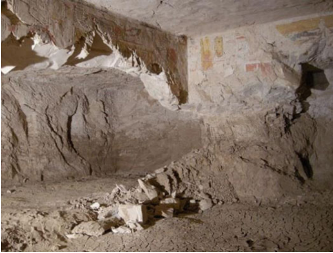
Fig. 1.3 Tomb of Nebattauy (QV60), Valley of the Queens, Luxor, Egypt, 19th Dynasty. Periodic flash floods have had a devastating effect on the expansive clay-rich limestone geology of the tombs in the Valley of the Queens, leading to catastrophic rock collapses and loss of painting, as shown here. Inherent geological issues at wall painting sites such as this often present problems that cannot be eradicated (© Stephen Rickerby )
