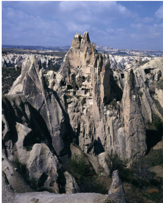
Fig. 3.7 a Virgin Mary Church in Göreme Valley. b Virgin Mary Church in Göreme Valley. Elevation mapping of the structural and macrostructural cracks that have occurred and still occur in the structure of rock churches and other surfaces remove
