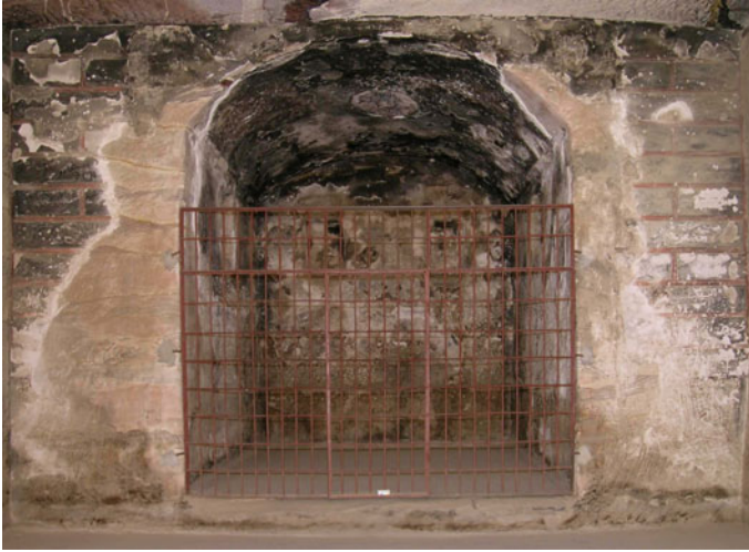
Fig. 5.2 The main chamber (the biclinium ) has two rock-cut benches, on its east and south sides, while a smaller vaulted recess is excavated in the back, south wall, as shown here. The biclinium 's south wall is decorated with painted stuccowork, which consists of an orthostat dado surmounted by fictive ashlar. The vaulted recess is painted in imitation of a bower heavily laden with ripened grapes. This image shows the cave complex before conservation (© Petra National Trust and Courtauld Institute )
