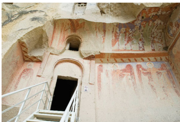
Fig. 4.45 Çavusin, Dovecote church, narthex. The ultramarine blue here is painted on a red background
