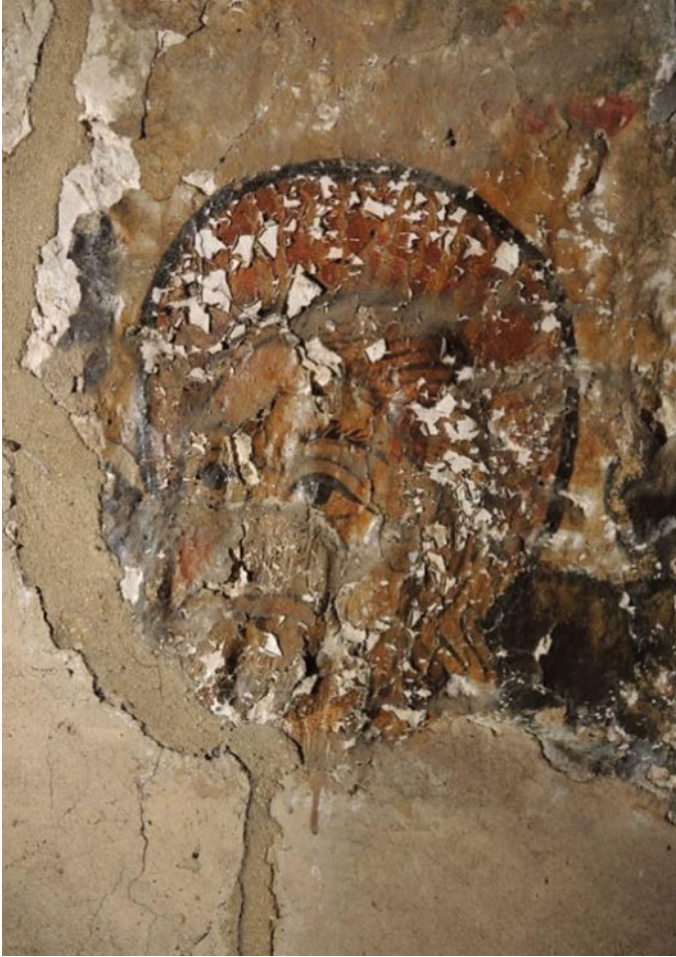
Fig. 1.5 Church of St Mary the Virgin, Cropredy, England, fifteenth century wall painting. This medieval wall painting was coated with an organic varnish, probably in the late-nineteenth or early-twentieth century, in an effort to preserve it. This has badly discoloured and is now promoting severe paint flaking and loss, as this detail shows. Wall paintings very quickly reach states of complete condition breakdown as a result of poor remedial treatment choices (© Stephen Rickerby )
