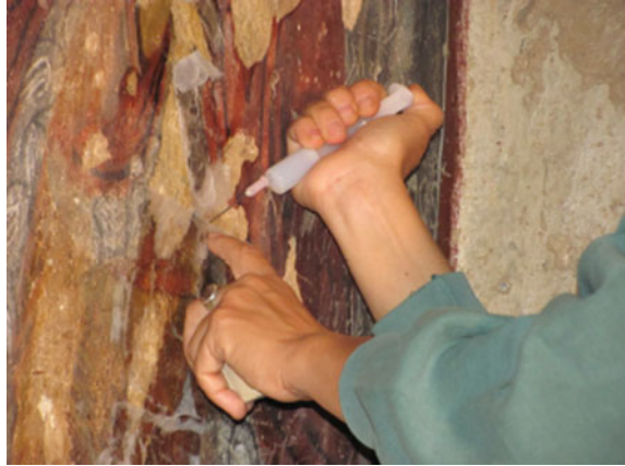
Fig. 3.13 In several churches, natural cracks caused by rain and frost eventually lead to separation and loss of important elements of the rock-cut surfaces. Specialist injection grouting is required, as shown here
