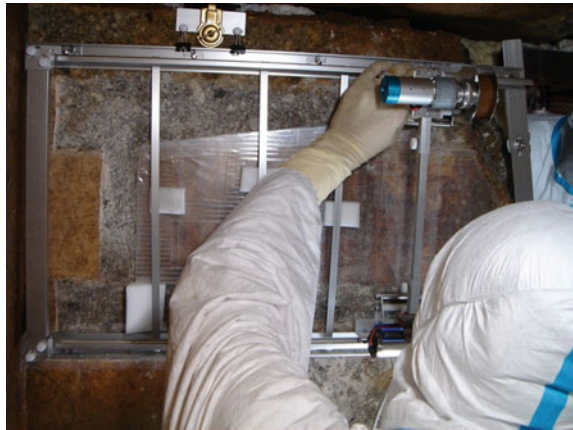
Fig. 16.10 Removing the painting of the Vermilion Bird from the Kitora tumulus with a diamond-wire saw
