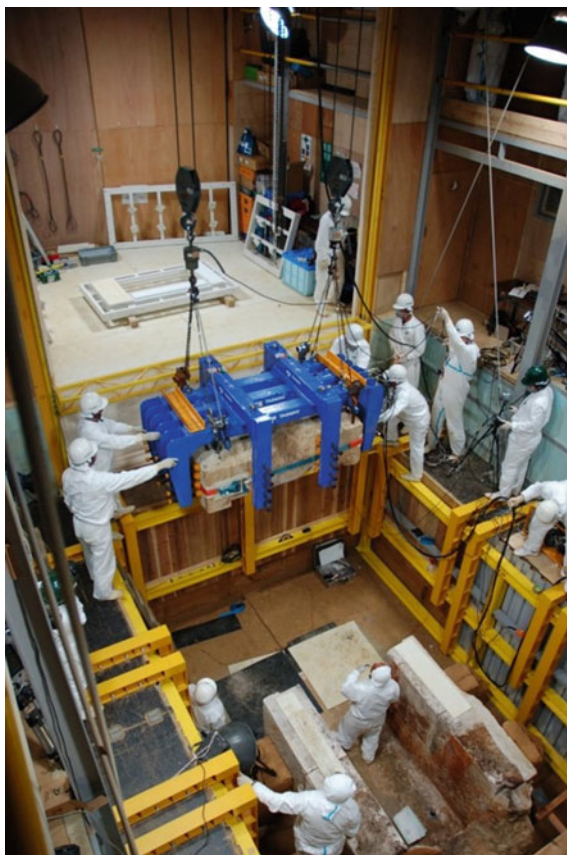
Fig. 17.4 Work to remove the ceiling stones
