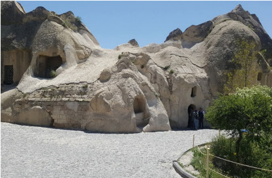
Fig. 3.12 a St. Basil Church, Göreme Open Air Museum. Before recent external treatment. The application of external renders to rock-cut churches in the past has not always been successful. b St. Basil Church, Göreme Open Air Museum, after external treatment
