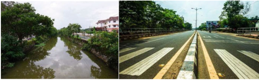
Fig. 10 Present condition of Sarovaram bypass
