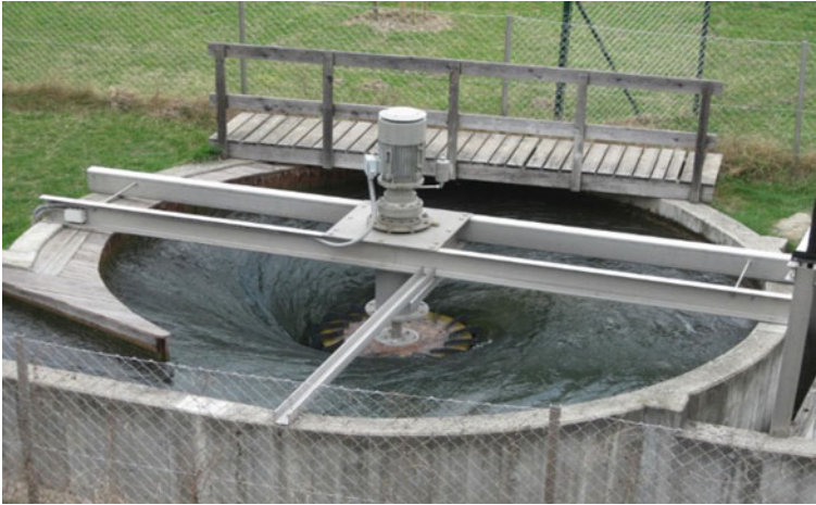
Fig. 1 Gravitational water vortex power plant [2]
