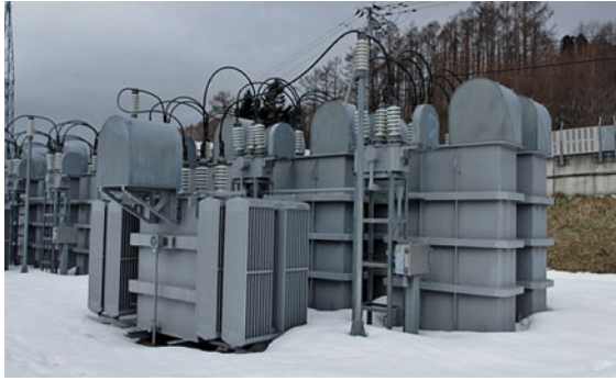
Fig. 8.23 Photograph of a 23 kV, 22.5 MVA shunt capacitor bank
