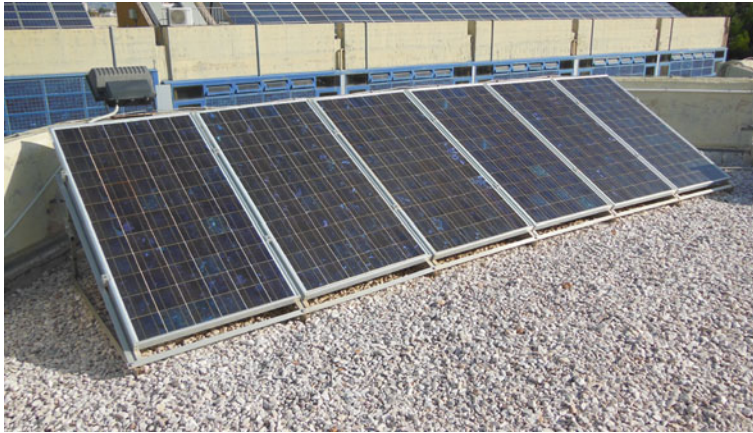
Fig. 15.11 A rooftop PV system installed at the Electric Energy Systems Laboratory of the National Technical University of Athens (Courtesy Authors)
