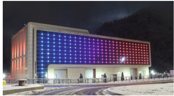
Fig. 11.21 The night lighting and facade of the Laura 110 kV Substation in Russia (Krasnaya Polyana—Sochi) is an example of design for aesthetics (Courtesy Electra)
