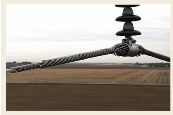
Fig. 9.107 Helically attached elastomeric suspension (adapted from [9.209])
