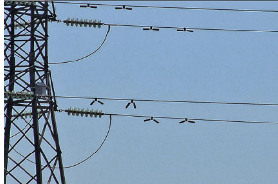
Fig. 9.169 Drooping vibration dampers (20 past 8 o'clock look)
