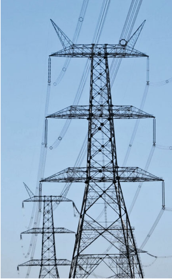
Fig. 9.4 1200 kV AC line at a test station in Bina, India (photo: A. Pigini)
