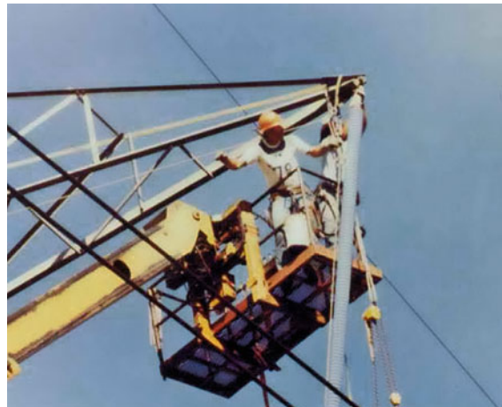
Fig. 9.179 Replacement of ceramic insulators with composite insulators (adapted from [9.269])
