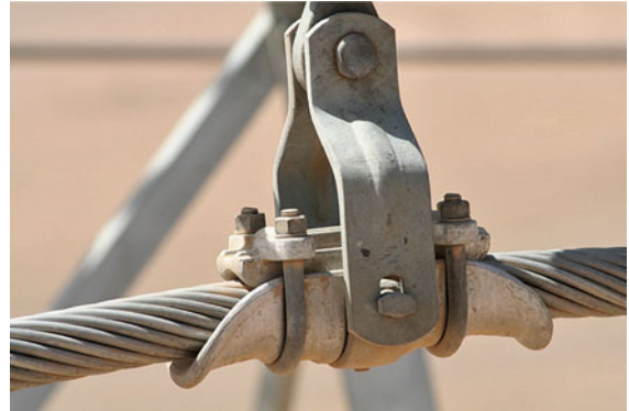
Fig. 9.105 Suspension clamp
