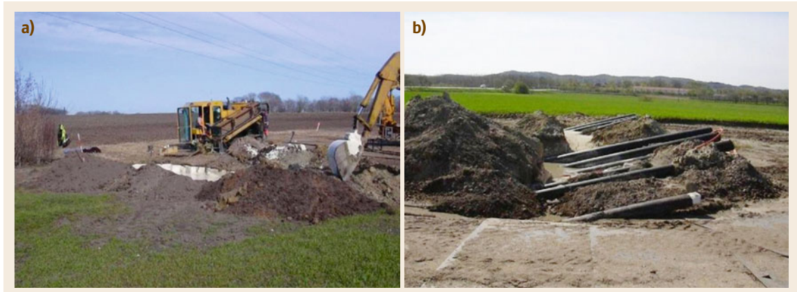
Fig. 10.13a,b Drilling machine (a) and pipes (b) for HDD (adapted from [10.17])
