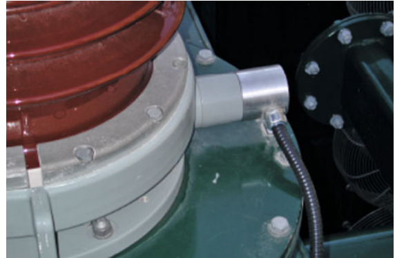
Fig. 8.137 Transformer bushing voltage sensor for application in a CSS. (Courtesy of Hydro Québec)
