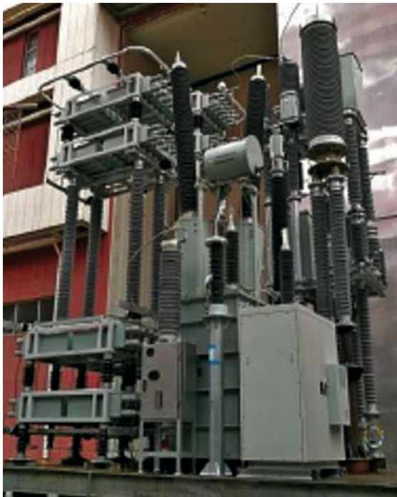
Fig. 8.165 Photograph of a 160 kV, 9 kA mechanical DC circuit breaker with current injection [8.81]
