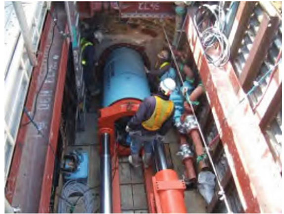
Fig. 10.104 Microtunneling in Japan (adapted from [10.14])
