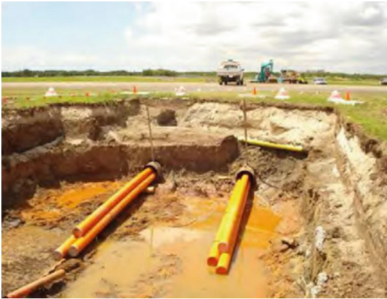
Fig. 10.98 Sleeve bore (adapted from [10.14])
