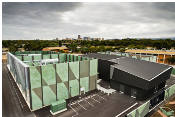
Fig. 11.1 City West Substation, Adelaide, South Australia (Courtesy Electranet)
