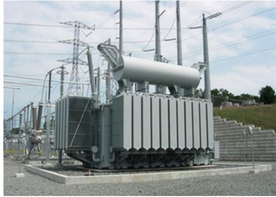
Fig. 10.52 Reactive compensator for a 30 km 345 kV PPLP pipe-type cable in the USA (adapted from [10.14])
