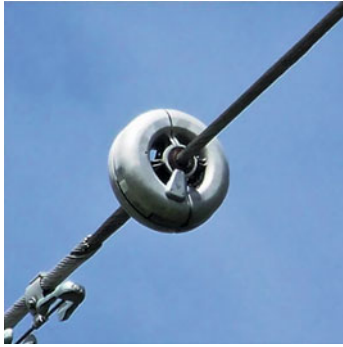
Fig. 9.45 Power donut (adapted from [9.96])
