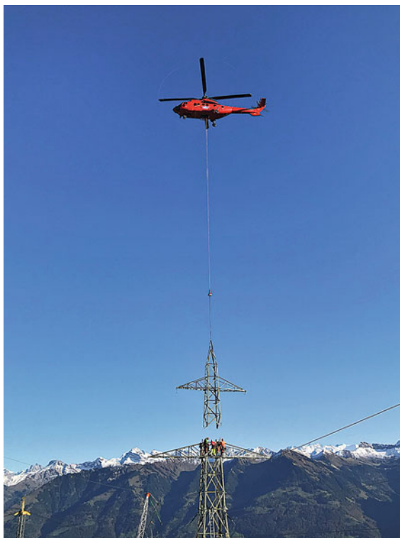
Fig. 9.163 Tower erection using a helicopter (photo Edward Steiner AG/CH)
