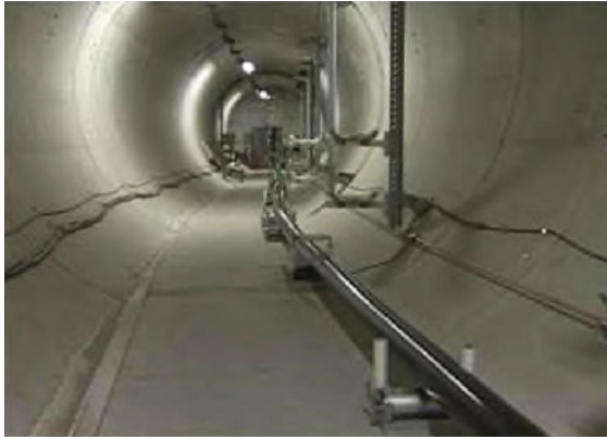
Fig. 10.108 Cable installation by motor-driven rollers in a tunnel (adapted from [10.14])
