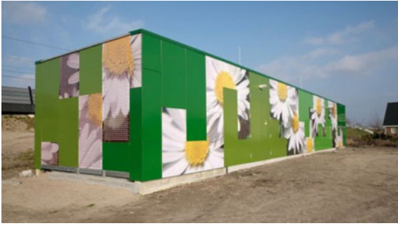
Fig. 11.24 Technical facilities with an attractive outer shell or fence in Dronten, Rotterdam, Liedsche Rijn, Utrecht (Courtesy Tennet)
