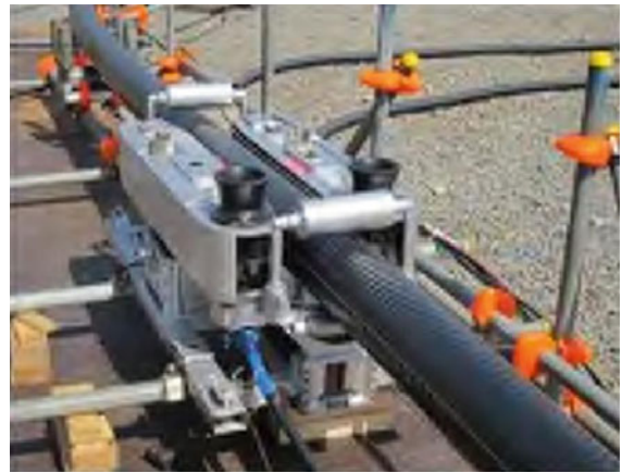
Fig. 10.109 Cable installation by a hauling machine (adapted from [10.14])
