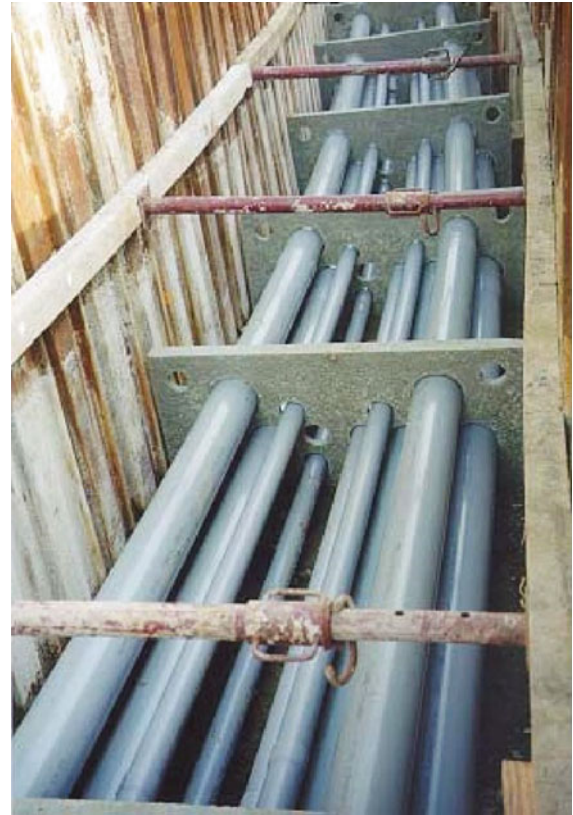
Fig. 10.10 Cables installed in ducts (adapted from [10.13])
