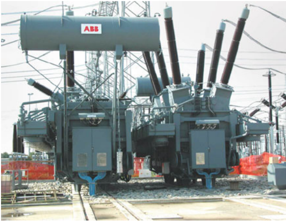
Fig. 7.88 Phase-shifting transformer [7.110]
