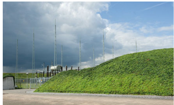
Fig. 11.22 Prinsenhage high-voltage substation in Breda Substation in the Netherlands (Courtesy TenneT/Movares)
