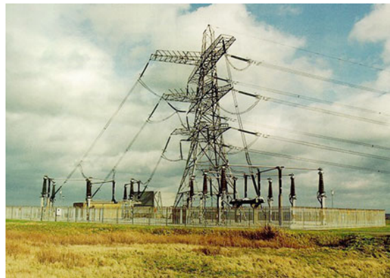
Fig. 10.6 EHV transition compound (adapted from [10.8])
