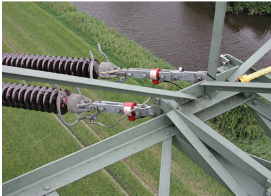
Fig. 9.46 Load cells (red) for tension monitoring (adapted from [9.96])
