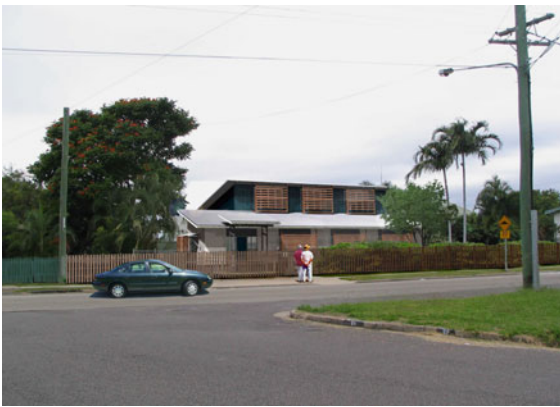
Fig. 11.25 3-D visualization showing a proposed new substation in a suburban street in North Queensland, Australia (Courtesy Ergon Energy)
