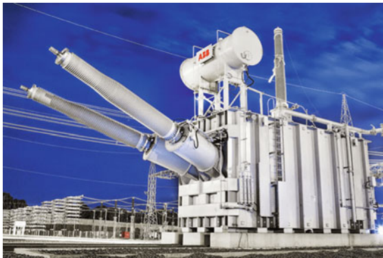
Fig. 7.91 800 kV HVDC transformer [7.111]
