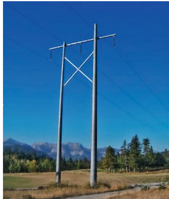
Fig. 9.142 FRP cross-braced H-frame
