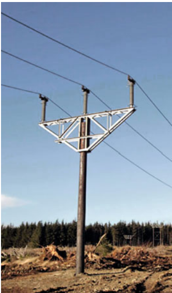
Fig. 9.67 Vertical post insulators in the so-called trident configuration (adapted from [9.112])
