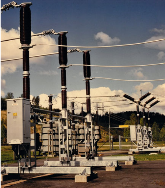
Fig. 8.36 245 kV, 50 kA double-break and single-break SF 6 puffer circuit breakers. (Courtesy of ABB, produced by ASEA)
