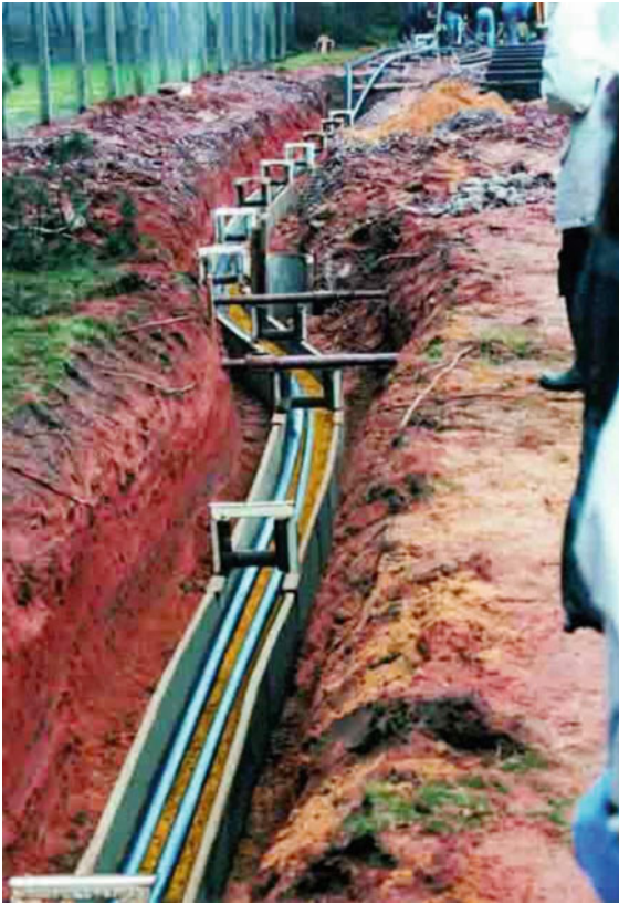
Fig. 10.11 Cables installed in troughs (adapted from [10.13])
