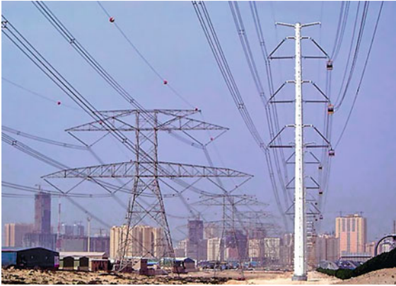
Fig. 9.151 Visual side-by-side comparison of conventional and compact 420-kV lines with the same power transfer capacity (adapted from [9.252])
