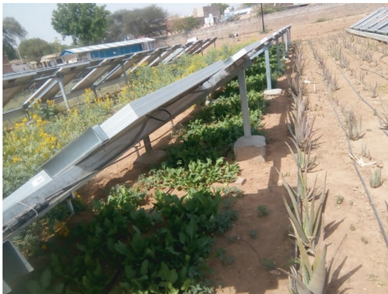
Fig. 11.13 Cultivation of spinach below PV module in agri-voltaic system. (Source: CAZRI Annual Report 2017–18, pp. 101–104)
