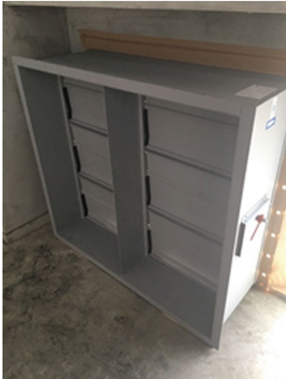
Photo 2 Differential pressure adjustment dampers
