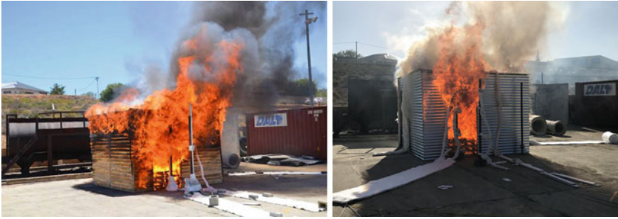
Fig. 8 Full-scale fire experiment on a timber clad shack (left) and corrugated steel (right)
