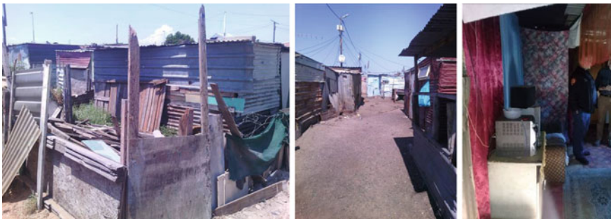
Fig. 2 Multiple shacks adjacent to each other (Left and middle). Note the timber pile, variation in construction types and materials of dwellings, and use of old and new materials, etc. Right-hand photograph shows a picture inside a dwelling where highly flammable materials are placed on walls for insulation, electrical appliances are present, and floors are carpeted or have a linoleum finish (such details vary from dwelling to dwelling)
