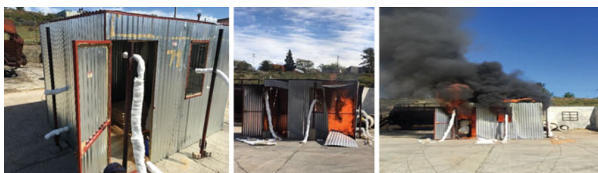
Fig. 4 Experimental shack setup (left), setup after the timber fuel load test (middle), and during the “representative” fire test (right)
