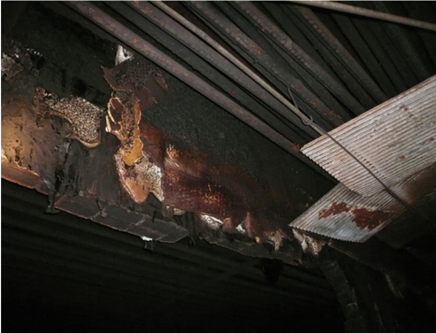
Fig. 2 Upper portion of the storage room
