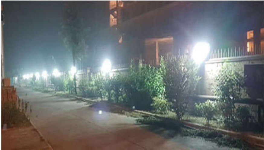
Fig. 2 Actual views of deployed G3-PLC based LED streetlight system
