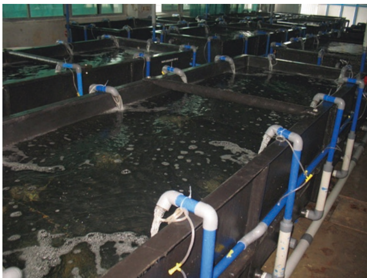
Fig. 10.6 Recirculating seawater system for broodstock maturation and rematuration of Thenus unimaculatus at Field Laboratory CMFRI, Kovalam, Chennai, India (Photo by: Joe K Kizhakudan, CMFRI)
