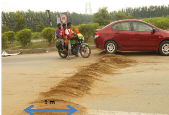
Fig. 6 Temporary speed breaker created on NH-58 in Muzaffarnagar. Source Author, July 2014, Muzaffarnagar
