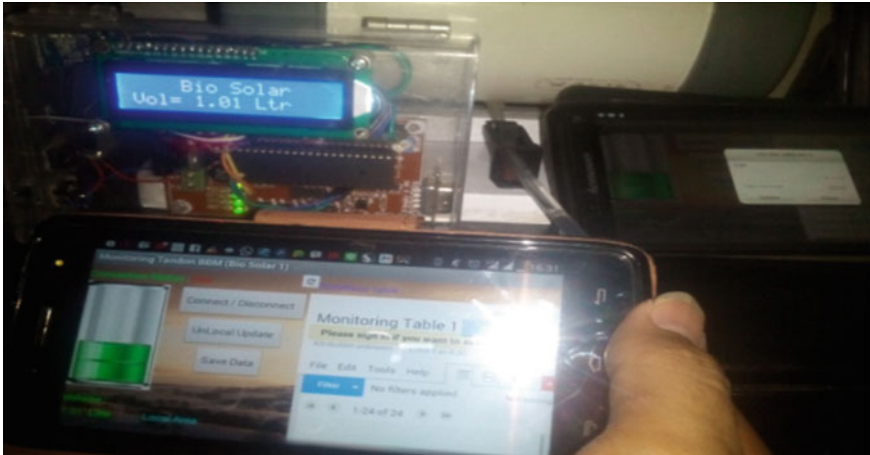
Fig. 76.6 Filling monitoring of 1 L via SMS gateway
