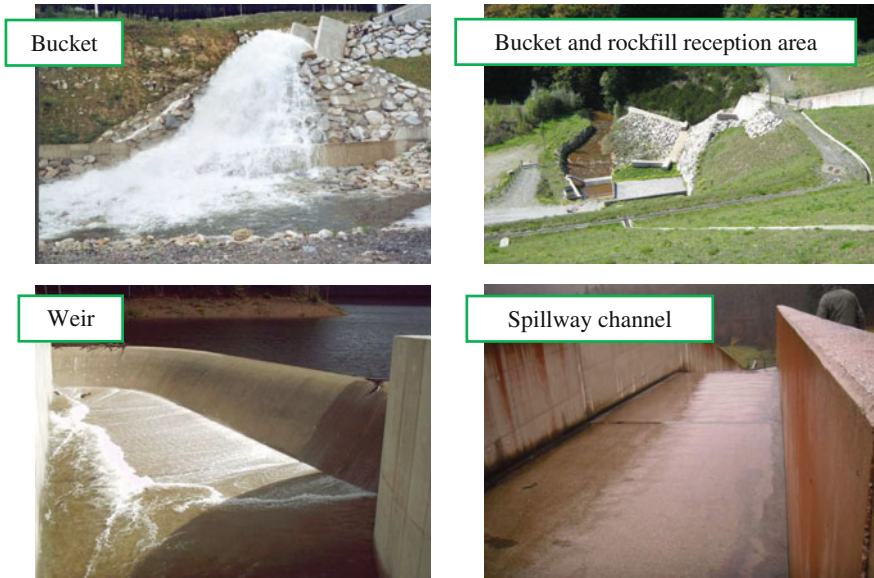
Fig. 3 Pictures of the spillway
