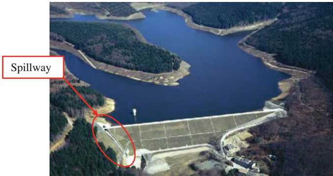
Fig. 1 The Galaube dam and the spillway
