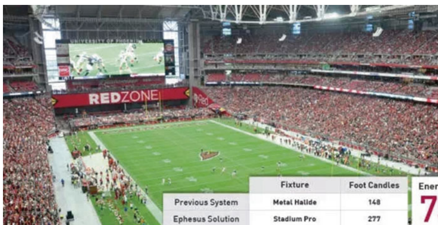
Fig. 11.2 LED lighting application (Source: http://www.ledinside.com.tw/news/20150203-30698.html )
