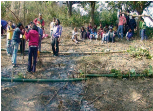
Fig. 18.6 Piling bamboos or firewood by a horizontal working method
