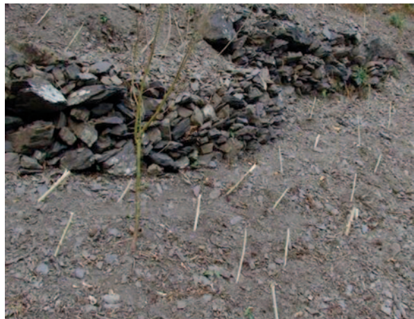
Fig. 18.5 Piling stones by a horizontal working method
