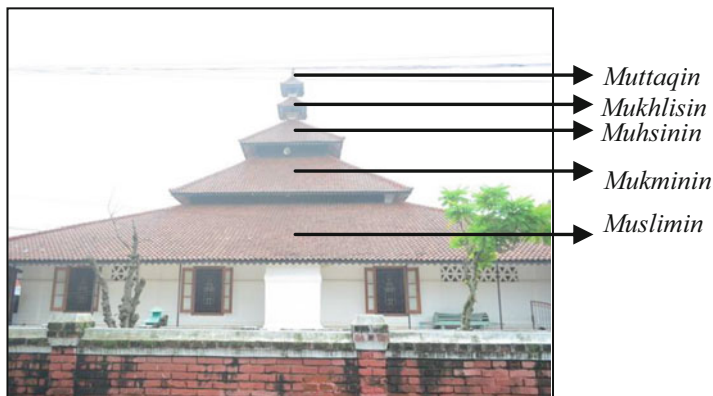
Fig. 17.1 The roof levels of the Banten Great Mosque representing characteristics of the Muslim
