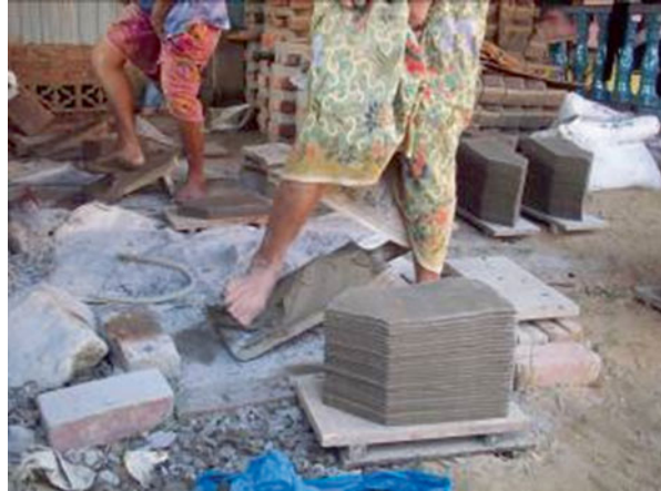
Fig. 66.3 The uniqueness of Singgora roof – kneading and forming using the legs
