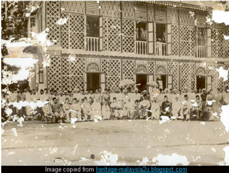
Fig. 54.1 Ihsaniah Iskandariah Mosque, Perak, Malaysia, in 1938. Its walls were made of woven hand cut bamboo strips and it had no minaret
