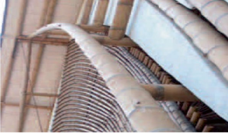
Fig. 54.4 Curve bamboos as column (courtesy of Simon Velez)
