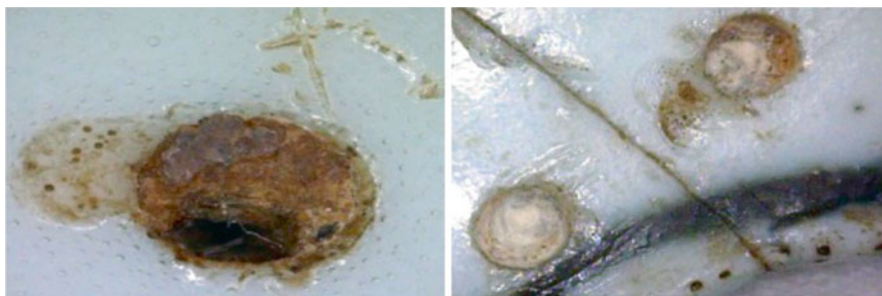
Fig. 13.4 The trace of holes from the removal of rivet, finding the damaged area and filler inside the holes
