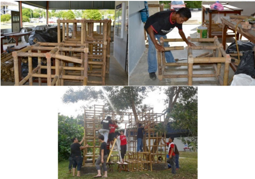
Fig. 54.17 Temporary Bamboo Workshop construction process at UiTM Perak involving activities with FSPU students, KUTAI UiTM Perak Academia, and the Design Principles Sdn. Bhd. The combined results of series bamboo modular cube designed are fundamental to the construction of this Bamboo Workshop
