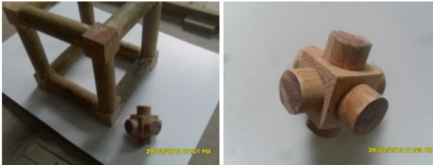
Fig. 54.16 The connector used in the system from wood material
