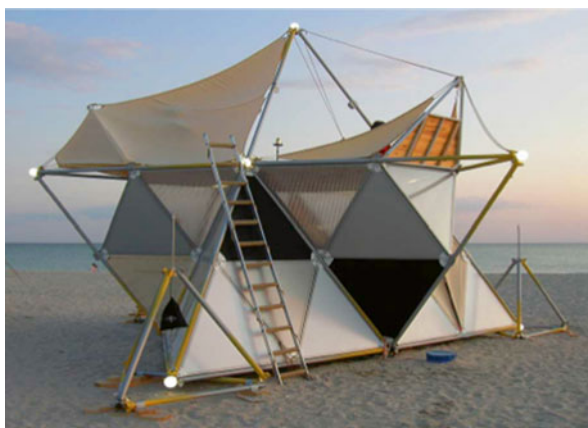
Fig. 54.8 A sophisticated triangulated structure strengthening the construction of mobile tent
