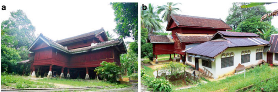
Fig. 28.3 (a, b) Shown are the architectural landscape elements and the concept of the Malay community garden at the Southern zone, Kg. Tanjong Penajis, Rembau, Negeri Sembilan (Source: Author, 2013)
