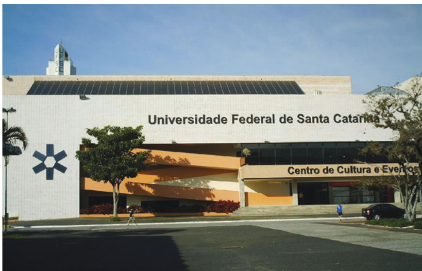
Fig. 7.7 Thin-film amorphous silicon (a-Si) rooftop PV system at the UFSC’s University Theater, in Florian  polis, Brazil (27  S latitude). The PV generator faces true North, and is tilted at 27  
