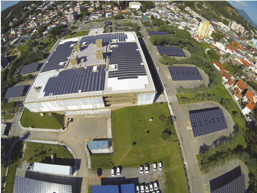
Fig. 7.11 Aerial view of the Eletrosul Megawatt Solar PV plant in Florianópolis, Brazil (27° South), showing the (450 kWp) rooftop and the nine parking canopies (565 kWp), which comprise the 1 MWp solar power plant
