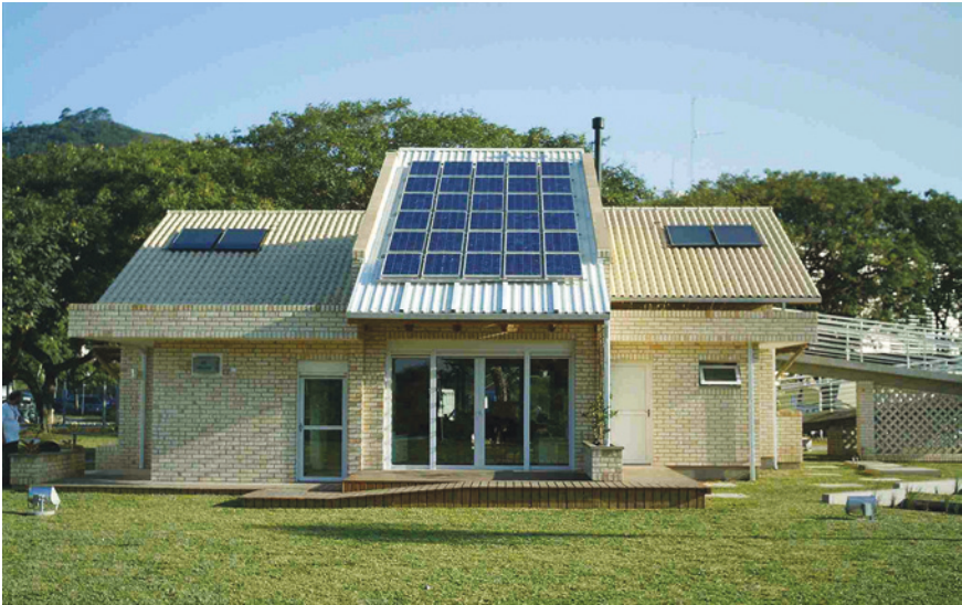
Fig. 7.6 Traditional crystalline silicon (c-Si) rooftop PV system at the Energy Efficient House, in Florianópolis, Brazil (27°S latitude). The PV generator faces true North, and is tilted at 27°
