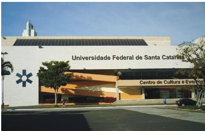
Fig. 7.7 Thin-film amorphous silicon (a-Si) rooftop PV system at the UFSC’s University Theater, in Florian  polis, Brazil (27  S latitude). The PV generator faces true North, and is tilted at 27  
